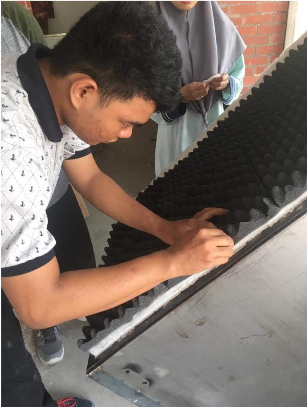
*Figure 3.3.4 Mounting the third layer of sound panel, acoustic foam.*
