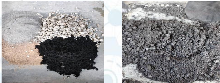
Figure 1: Mix concrete for slump test
