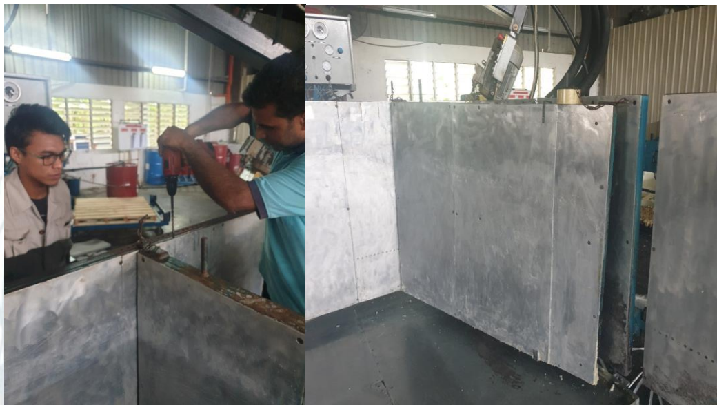
Figure 3 The fabrication and installation of the fixture
