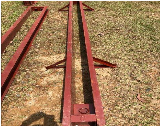
Figure. 5. Roof beam Steel Formwork
