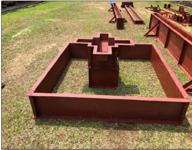
Figure 11. Pad Footing Steel Formwork
