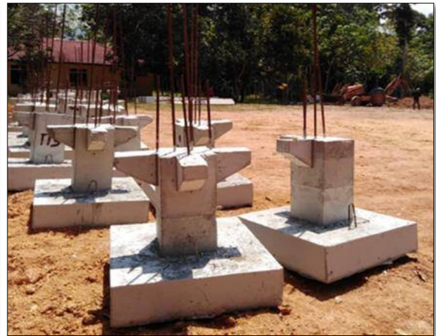
Figure 12. IBS Pad Footing
