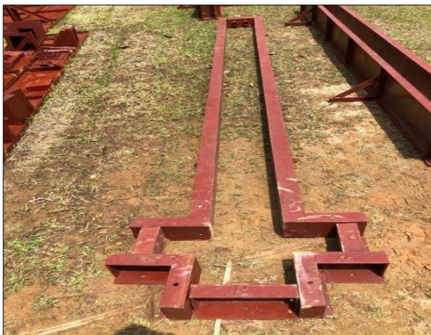
Figure. 3. Column Steel Formwork
