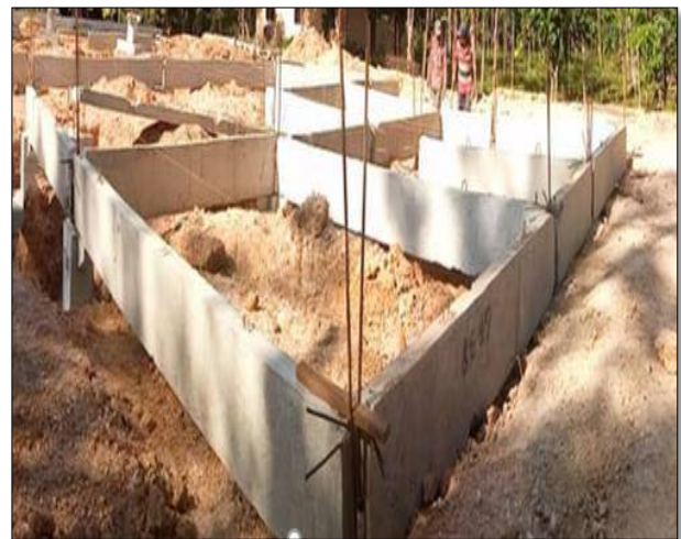
Figure. 8. IBS Ground Beam
