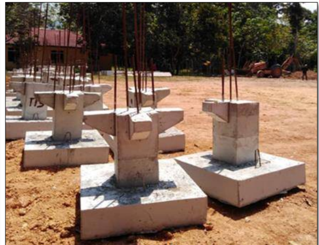
Figure 12. IBS Pad Footing
