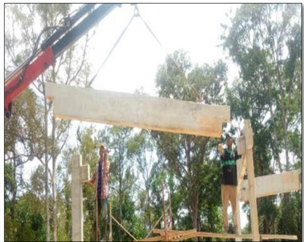
Figure. 6. IBS Roof Beam
