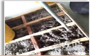
Put the mixture into the mould and tamped using tamping rod
