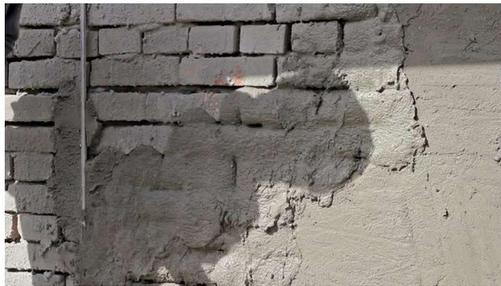
Figure 1: Cement-sand brick wall and plastering
