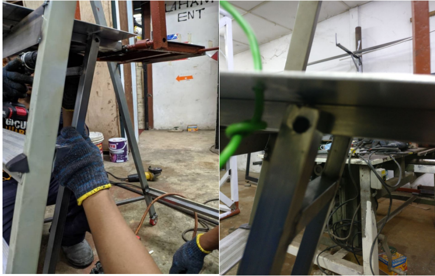
Figure 3.2 Installation of ‘ Supporting Leg ’
