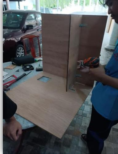
**the process of joining between pieces of play wood using screws.**
