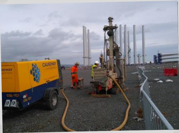
Figure 16 : Rotary Coring
