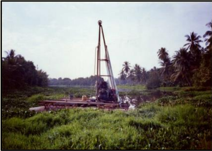
Figure 5 : Standard Penetration Test for Bridge Project
