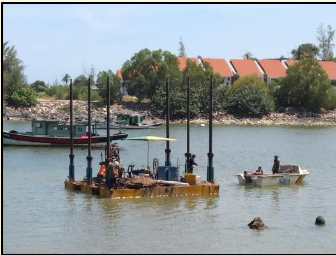
Figure 6 : Standard Penetration Test for Jetty Project
