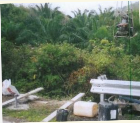
Figure 8 : Movement of boring machine Using Mobile Crane
