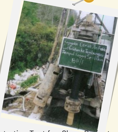
Figure 7 : Standard Penetration Test for Slope Project
