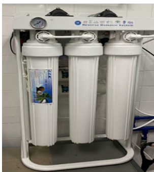
Figure 5: The RO filter supply for the tank
