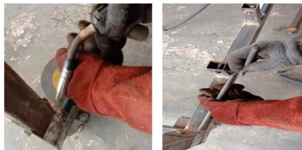
Figure 3.16 The process of installing the sub roller
