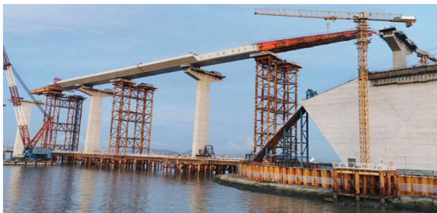
Fig. 8 Large section jacking of steel box girder
