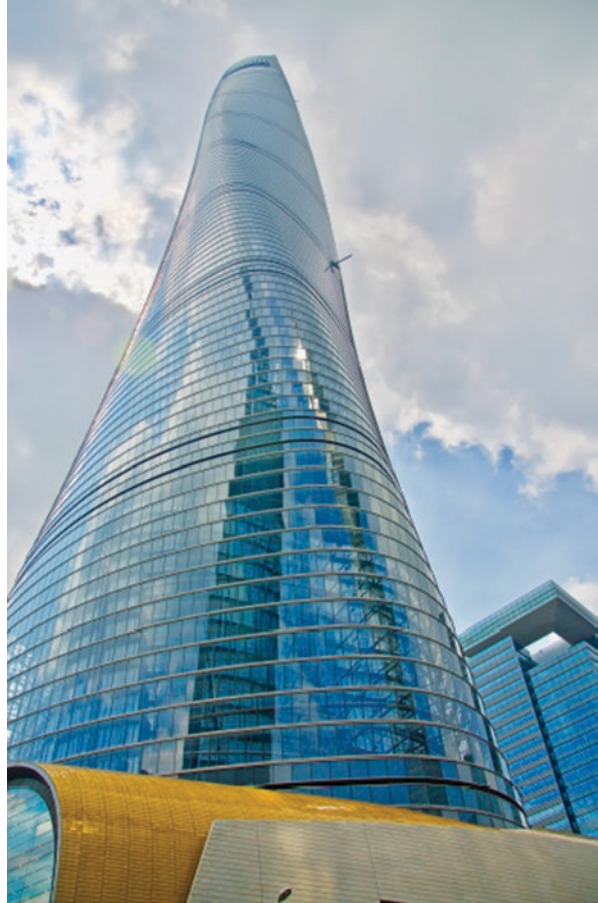
Fig. 12.1 Shanghai Tower, China – nine cylindrical buildings stacked atop each other with innovative double-layered facade twisting as it rises to reduce wind loading
