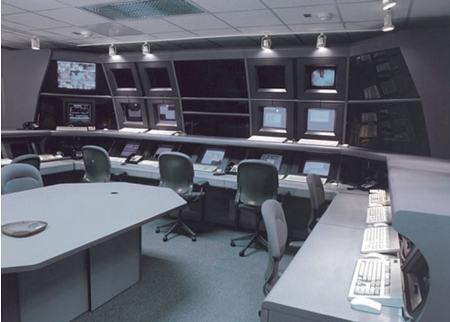
Fig. 17.4 Example of a fire/security command center (Photo by Jensen Hughes)
