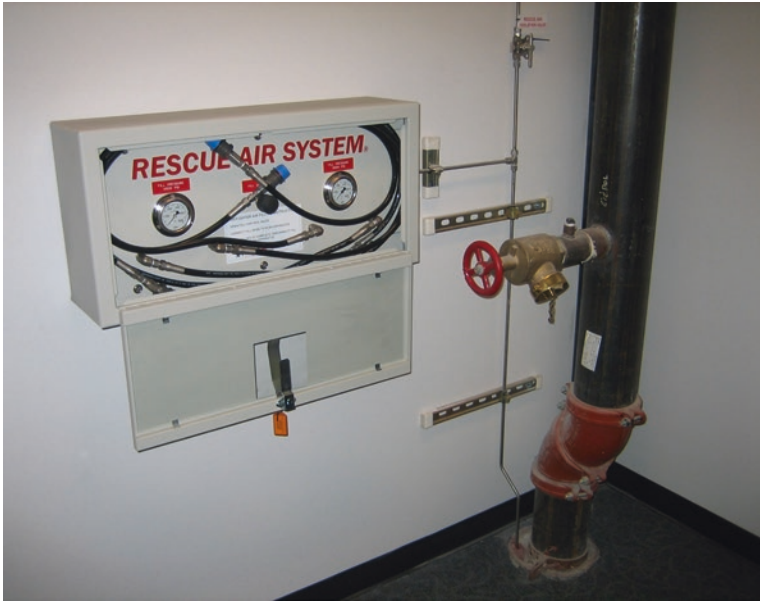
Fig. 17.3 Fire fighter air refilling station located inside a stairway, photo by Joe McElvaney
