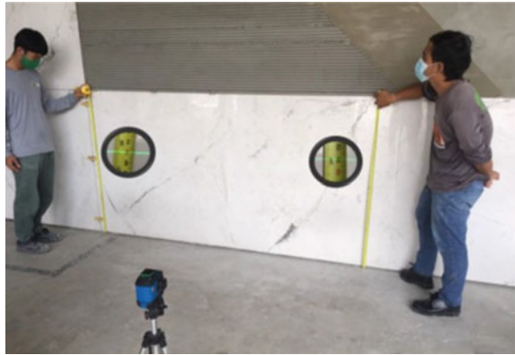
Fig. 2 Slope measurement on site
