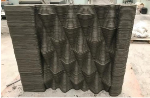
Fig. 6 P01 type 02 wall when finished construction
