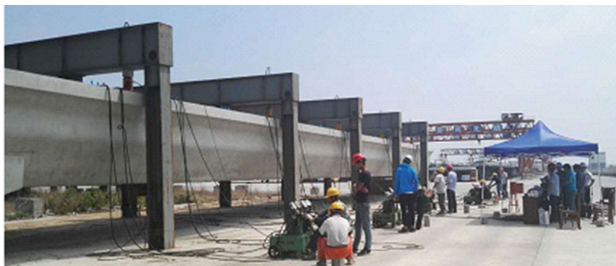
Fig. 4 Site of test
