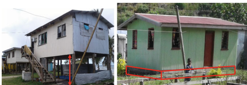
Fig. 7 Timber-framed houses on stilts (left) and a concrete foundation (right). Source ElkhARBoutly [13]
