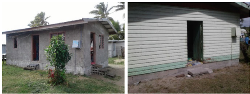
Fig. 12 Concrete houses on a concrete foundation, with two courses above the ground being common practice. Source ElkhARBoutly [13]
