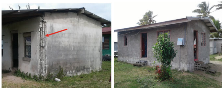
Fig. 8 Concrete-block house with reinforced columns (left); a concrete-block house without steel reinforcement (right). Source ElkhARBoutly [13]
