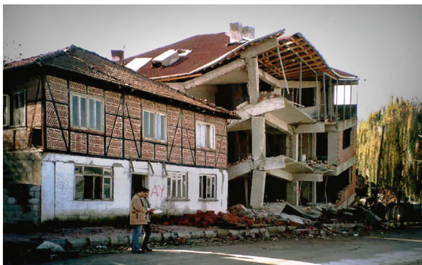
Fig. 5 Traditional Himis building standing while modern reinforced concrete building collapsed during 1999 Düzce earthquake [15]
