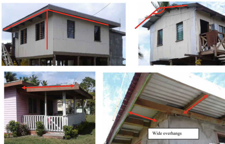
Fig. 9 Flat roof (top left); gabled roof with exposed eaves (top right); large roof overhang (bottom left); flat roof with wide eaves (bottom right). Source Elkharboutly [13]
