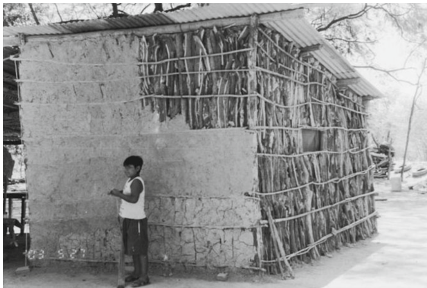
Fig. 9 Under construction Quincha house with wood and clay walls [11]
