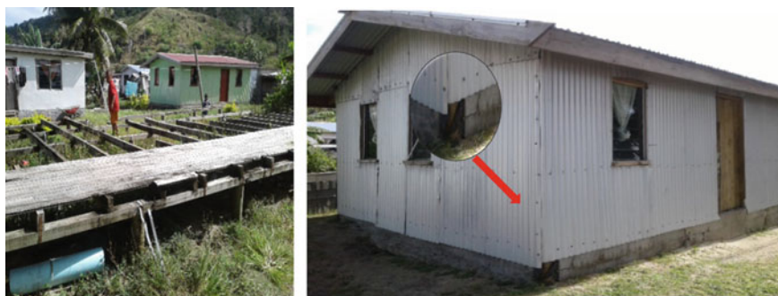
Fig. 6 Concrete foundation with timber corner post embedded into the foundation (left); damaged raised timber platform (right). Source ElkhARBoutly [13]
