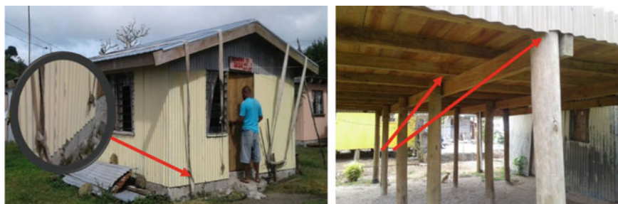
Fig. 10 Locals attempting to strengthen the roof structure (left); a house's structural connection with no metal straps (right). Source Elkharboutly [13]
