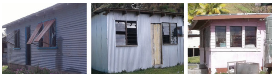
Fig. 14 Windows protected with timber shutters (left); unprotected louvred glass windows (middle); steel-mesh-protected glass windows (right). Source ElkhARBoutly [13]
