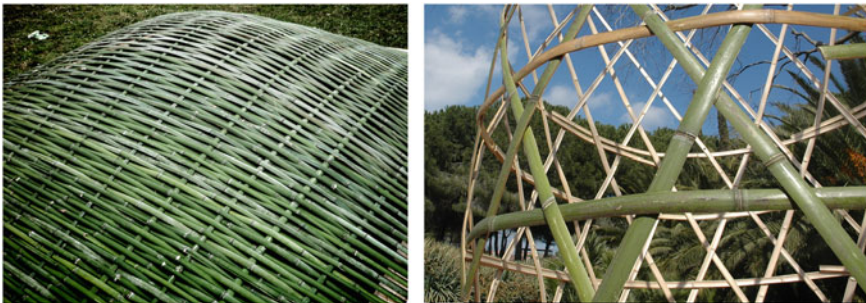
Fig. 6 Woven shells with bi-axial (left) and tri-axial (right) patterns
