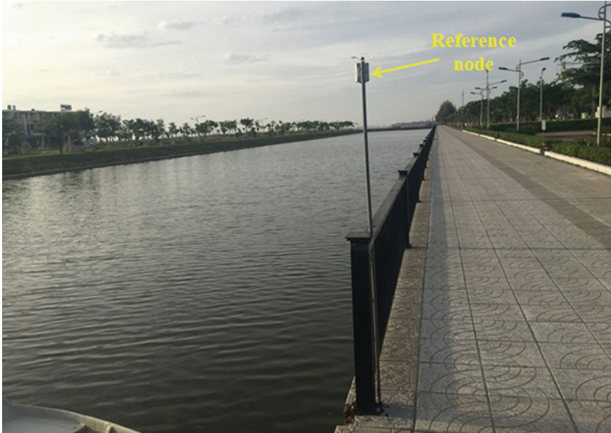
Fig. 6 Installation of Reference nodes at river bank
