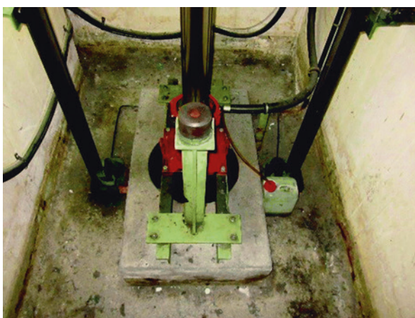
Fig. 6.19 Direct hydraulic lift, suspension 1:1. (Source: Author)
