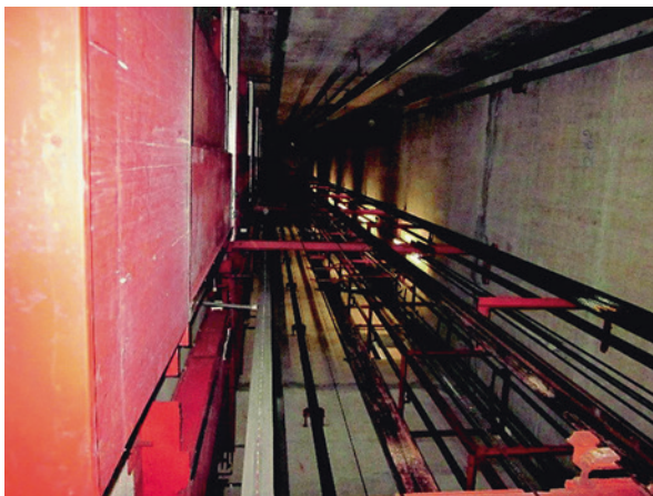
Fig. 3.5 Lift well from inside (Source: Author)
