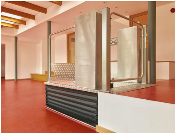
Fig. 4.7 Wheelchair lift with a swinging door at the end of the upper landing. (Source: HIRO Lift®, Bielefeld, Germany)
