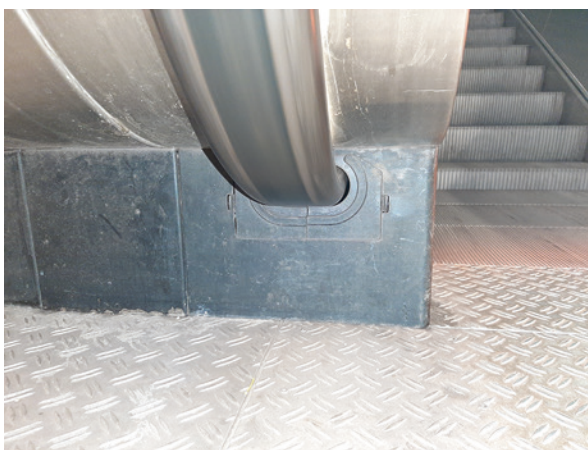
Fig. 28.28 Handrail insertion at the landing site below the balustrade. (source: author)
