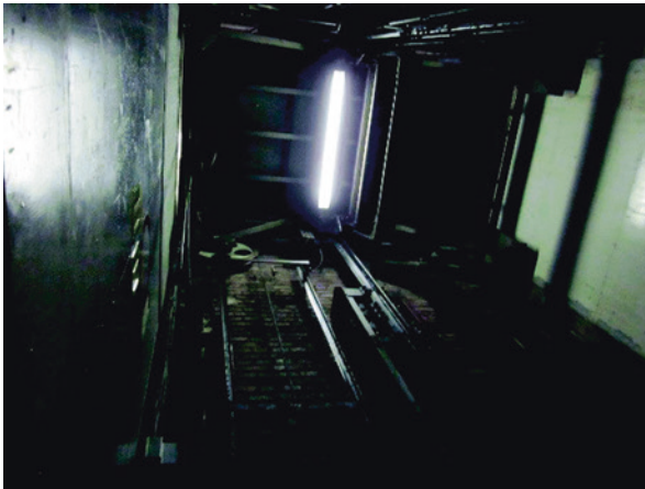
Fig. 6.25 Support chain with counterweights. (Source: Author)
