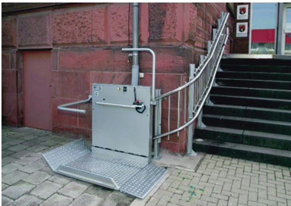
Fig. 4.22 Outdoor inclined wheelchair lift. (Source: HIRO Lift®, Bielefeld, Germany)
