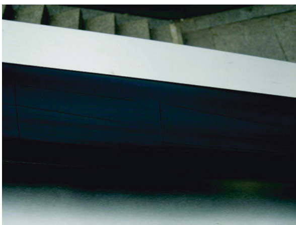
Fig. 32.2 Vandalism damage to a handrail. (Source: Author)
