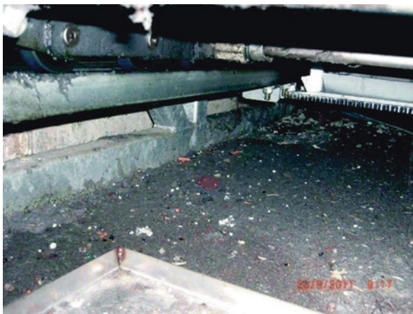
Fig. 31.1 Fluff formation in the step band system. (source: author)
