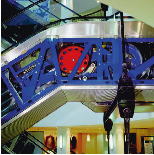
Fig. 28.1 Escalator tower (blue) with handrail drive wheel (red) (Source: Schindler Deutschland AG & Co. KG, Germany)
