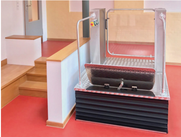
Fig. 4.6 Wheelchair lift for bridging stairs. A barrier at the lower landing serves as a closure. (Source: Liftwerk GmbH, Kaufungen, Germany)
